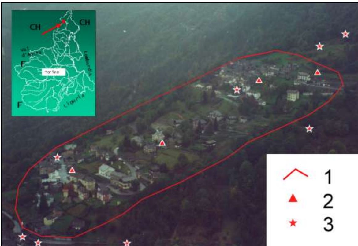
Fig. 56: The Graniga ridge in Bognanco. Legend: (1) High risk area in accordance with National Law. (2) Inclinometers. (3) Main slides, mudflows and fractures developing during heavy rains.
