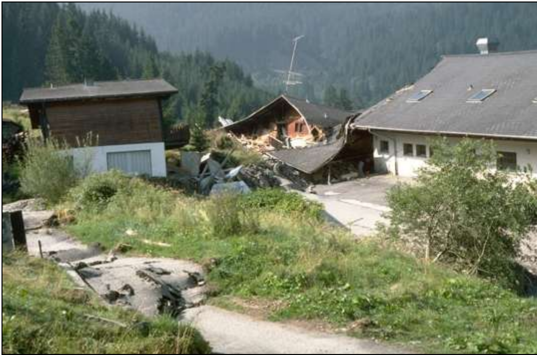
Fig. 1: Reactivated landslide Falli Hölli, CH. Total destruction of the village in June 1994
